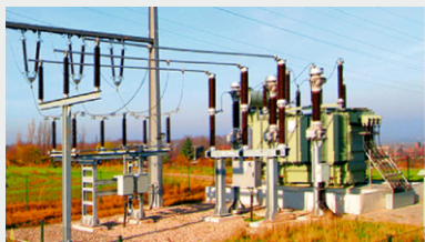
33KV/66KV Switch Yard
